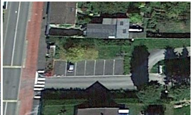
Parking centre de La Trugalle
